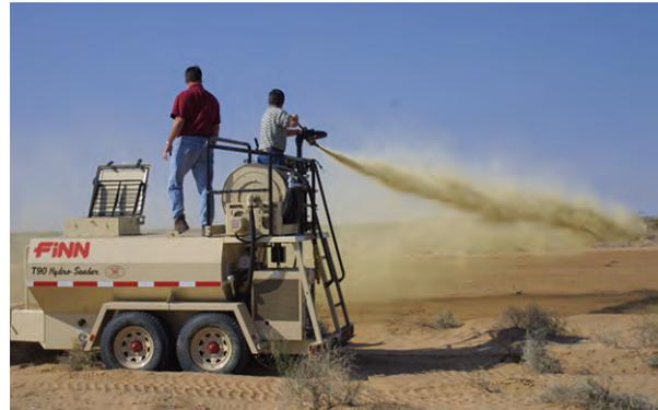
Photo 6. Distributing emulsion onto helipad using tower gun
