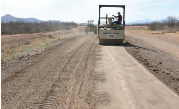
Photo 11. Compacting road surface after tilling (step *g*)
