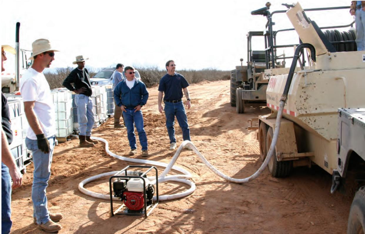
Photo 31. Transferring dust palliative from container to hydroseeder with centrifugal pump
