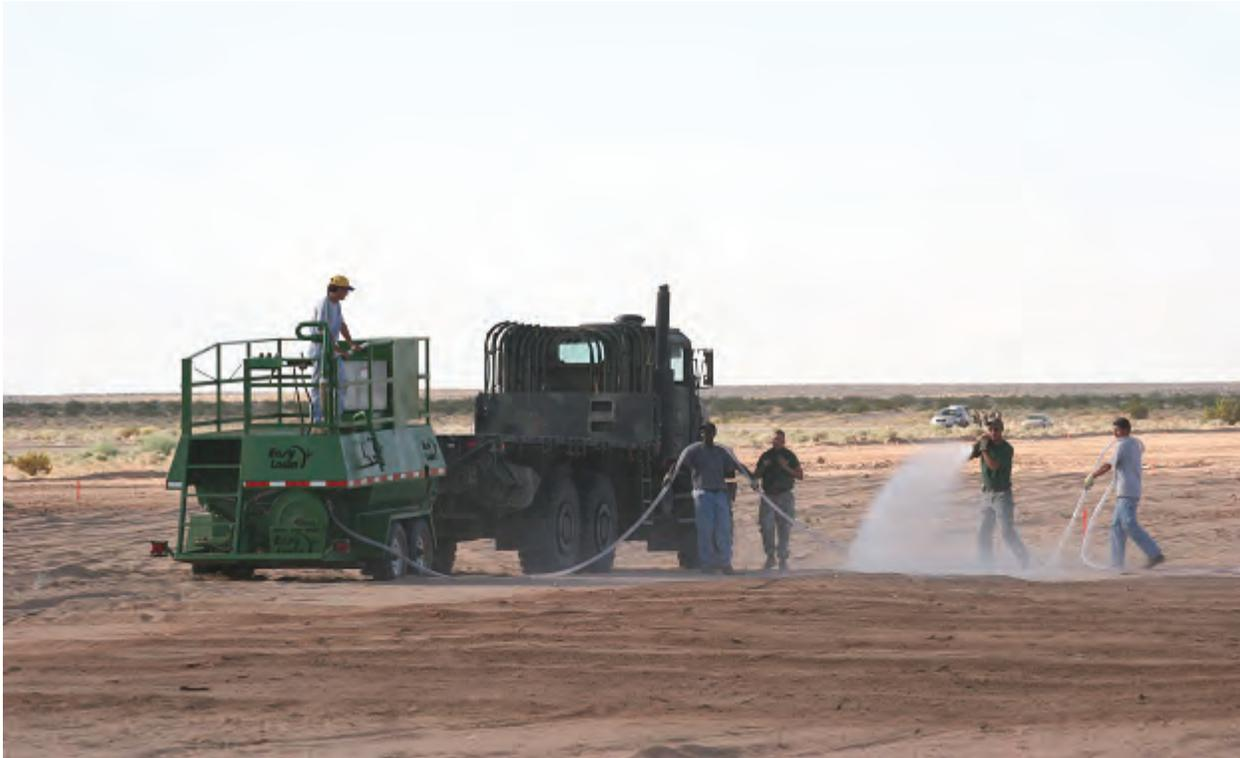
Photo 16. Treating heliport using hand-held hose on Easy Lawn hydroseeder
