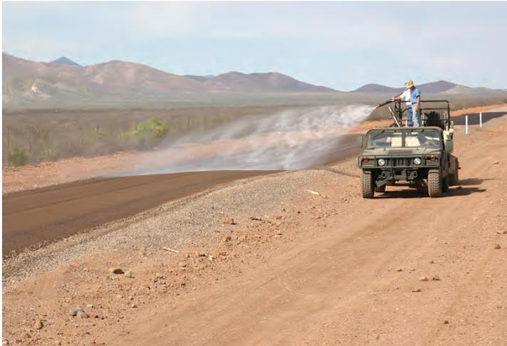
Photo 13. Applying synthetic fluid to road surface using wide-fan nozzle on tower hydroseeder
