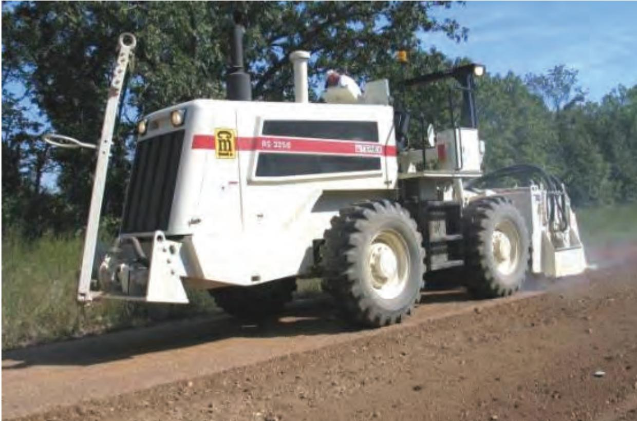
Photo 30. Mixing dust palliative in soil with rotary mixer
