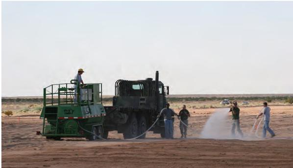
Photo 3. Spraying helipad using hand-held hose
